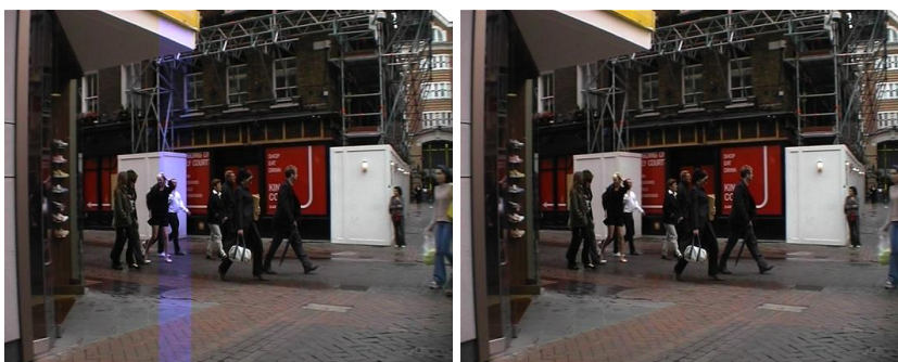
Figure 18.2 Damaged frame. Figure 18.3 Repaired frame.
