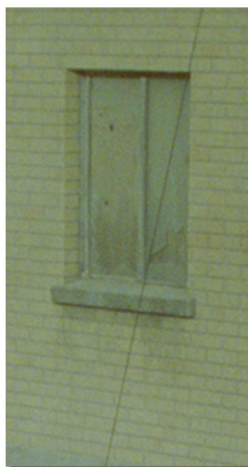
Figure 35.9 Cropped image of a wire across a brick wall/
