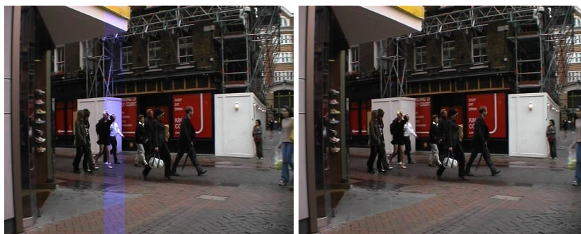
Figure 22.4 Damaged frame. Figure 22.5 Repaired frame.
